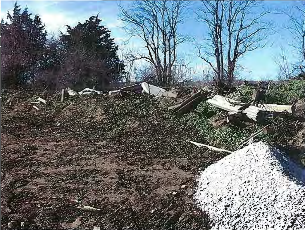
Date:01-30-2012 Time: 12:02PM Direction: Southwest Photo by: Jen O'Hearn Exposure #: 003 Comments: View of dimensional lumber, landscaping timbers, metal rebar, concrete, etc. on ground.
