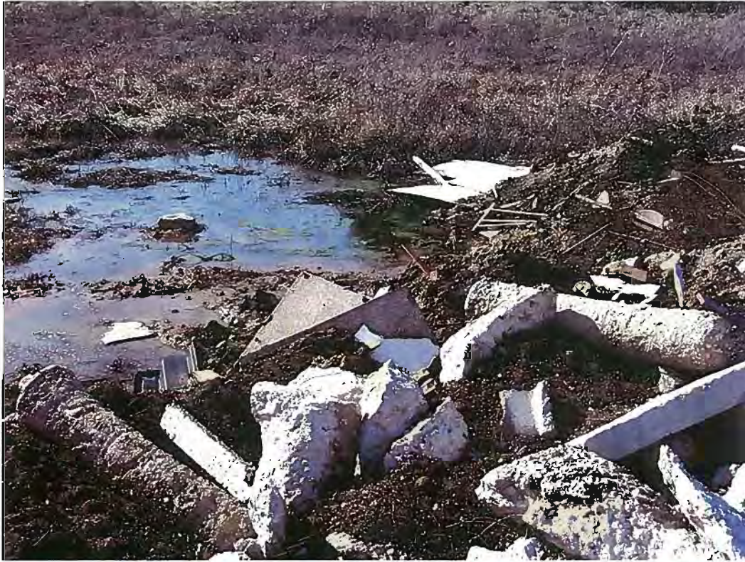
Date:01-30-2012 Time: 12:03PM Direction: Southwest Photo by: Jen O'Hearn Exposure #: 005 Comments: View of black plastic partially buried and along water area, plywood and dimensional lumber along water area, a piece of drywall, several pieces of concrete and concrete around pipe, etc.
